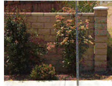
SPLIT FACE BLOCK WALL WITH CAP AND SPLIT FACE PILASTER WITH PRECAST CAP TO MATCH EXISTING ADJACENT COMMUNITY WALL
